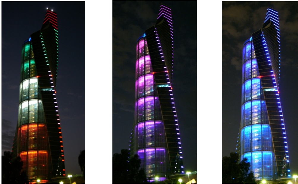
Figures 4 a, b, c: Al-Tijaria Tower, Kuwait. A recently completed KSLD project demonstrating use of DMX controlled colour changing LEDs; one scene is linked to wind-speed, with windier conditions causing lit bands to extend further down the facade.
